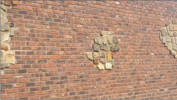
Stonework mixed in with the brickwork
